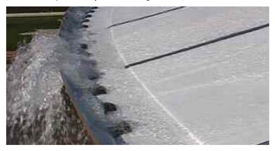
The immediate cause of the incident at Buncefield was put down to failures in level instrumentation and in the overfill protection safeguarding systems. The hardware failures were exacerbated by multiple systematic failures in the design, installation, operation, maintenance and testing of safety systems.
