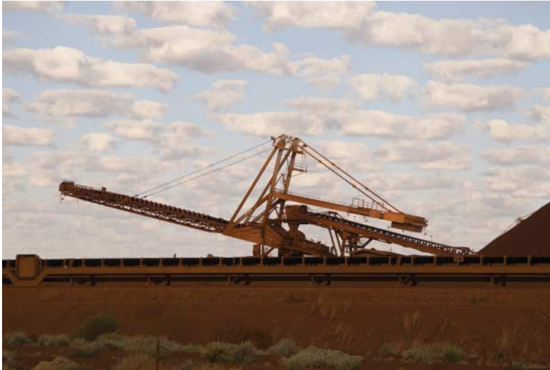
Figure 2. Stacker Conveyor. Source: Reproduced with permission.
